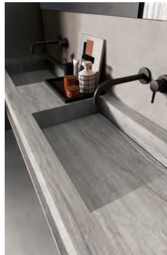
wall CONCREA PLAIN SILVER integrated top with 2 washbasins and washbasin top HORIZON SMOKE floor CONCREA PLAIN SILVER
